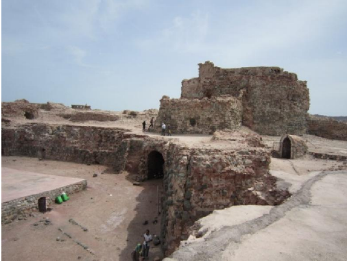
Figure 13: internal façade of the Portuguese Fortress
