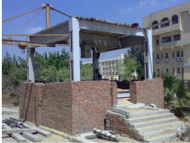
Fig (7) Soil chamber and loading frame
