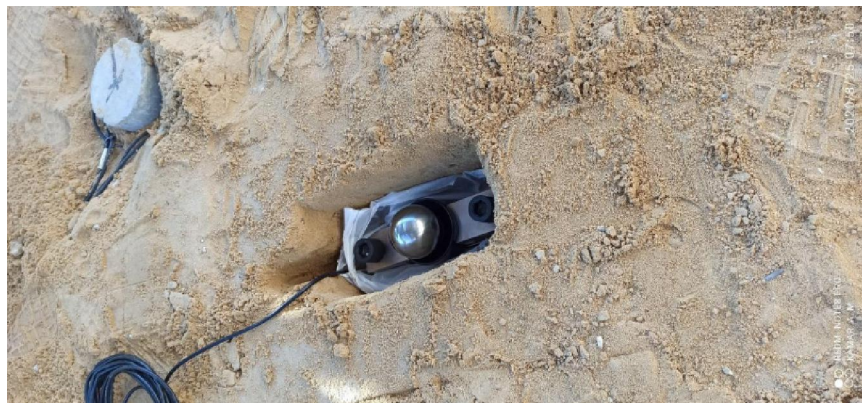
Fig (14) Placing load cell under the cap - group of four piles
