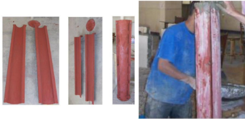
Fig (3) Description of forms and Casting of piles
