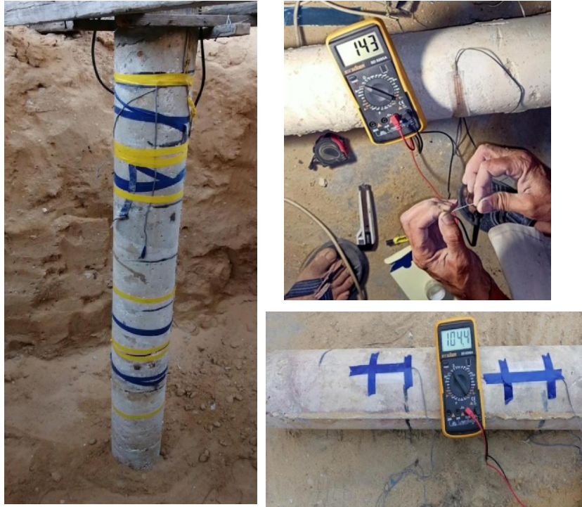
Fig (6) strain gauges installation on concrete piles
