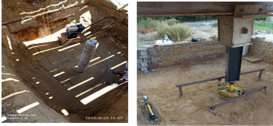
Fig (12) Mechanical compactor and setup for group (1) – (single pile)
