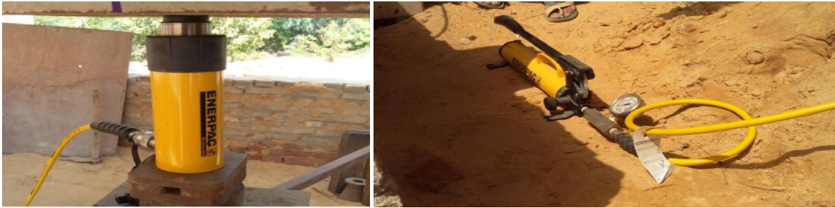
Fig (8) Loading jack and pump
