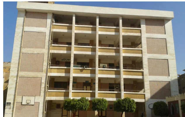
Picture.1 for EL-Wasta Prep School, source researcher
