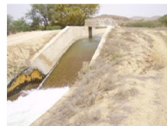
Figure 14: 170 CUSEC Water from Hub Dam to Main Canal Proposed Site for MHPP-2
