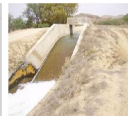
Figure 19: Site for Civil Work for Raising Water Head for MHPP-2 and MHPP-3
