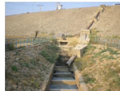
Figure 12: Water from Hub Dam to Main Canal Proposed Site for MHPP-1
