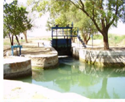
Figure 7: Bifurcation to Karachi and Lasbella through Manually Operated Gates
