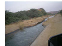
Figure 15: 150 CUSEC Water from Hub Dam to Main Canal Proposed Site for MHPP-3
