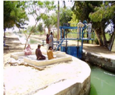
Figure 9: Operating of Manual Gates from Controlling Water Supply
