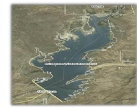
Figure 4: Aerial View of the Hub Dam
