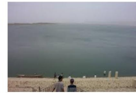
Figure 2: The Hub Dam Storage
